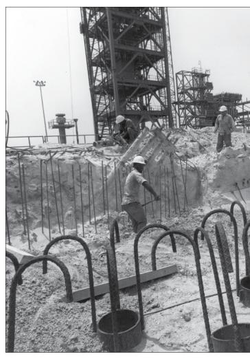
Looking like a giant erector set, Launch Pad 39A underwent major renovation in the I 970s to evolve it from the Apollo era 'clean' pad to include more fixed structures to support Space Shuttle launches.
